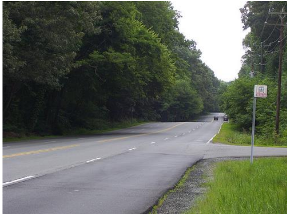
Figure 58: Lawyers Road Before Road Diet/VDOT
