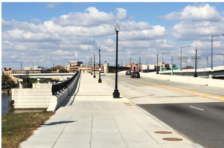
Figure 37: 11th Street Bridge/TPB/Michael Farrell
