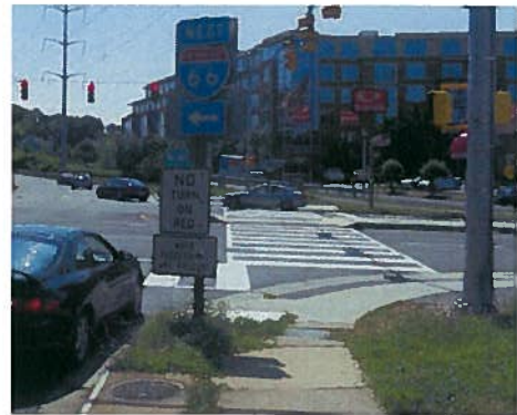
Figure 16: Location of Existing Signs Block View of Trail
