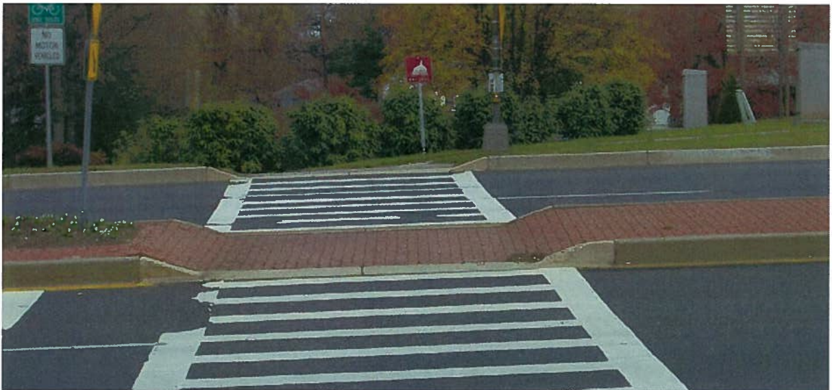
Figure 11: Example of widened median with full width curb cut and differentiating surface treatment
