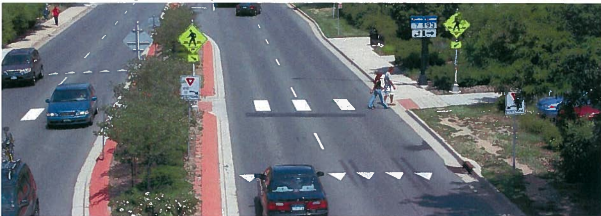
Figure 6: Example of an advanced yield line utilized in conjunction with a Rapid Flashing Beacon installation in Boulder, CO
