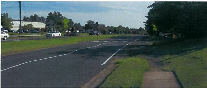
Figure 9: It is recommended to trim existing vegetation and complete the sidewalk connection to the trail in addition to providing advanced yield line and rapid flashing beacons
