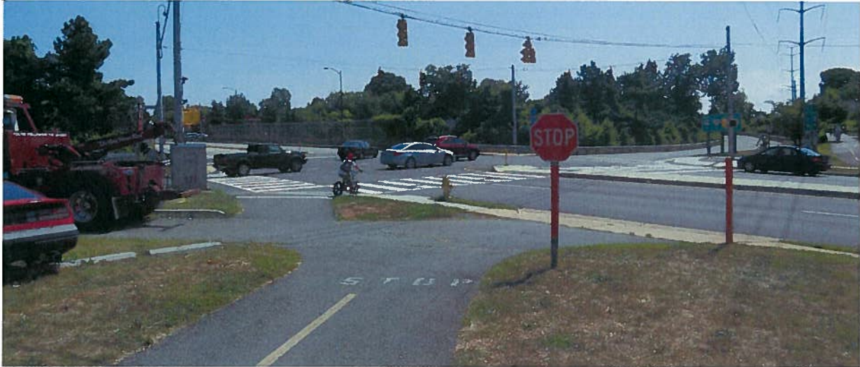
Figure 17: The existing approaches to Lee Highway do not clearly define the primary trail alignment to the user. The driveway should be subservient to the trail at this location with some wayfinding signs provided to guide the user towards the crosswalk for the trail/Metro Station or alternatively to Lee Highway via the driveway.
