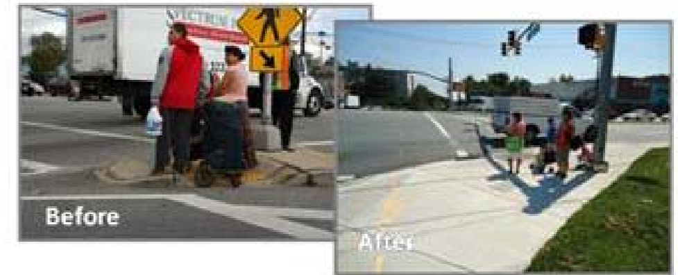
MDSHA Piney Branch Road & University Blvd Intersection Improvements (2009)
