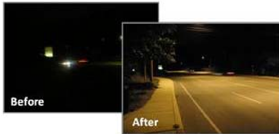
Lighting Improvements: University Boulevard to PGC Line (2011)
