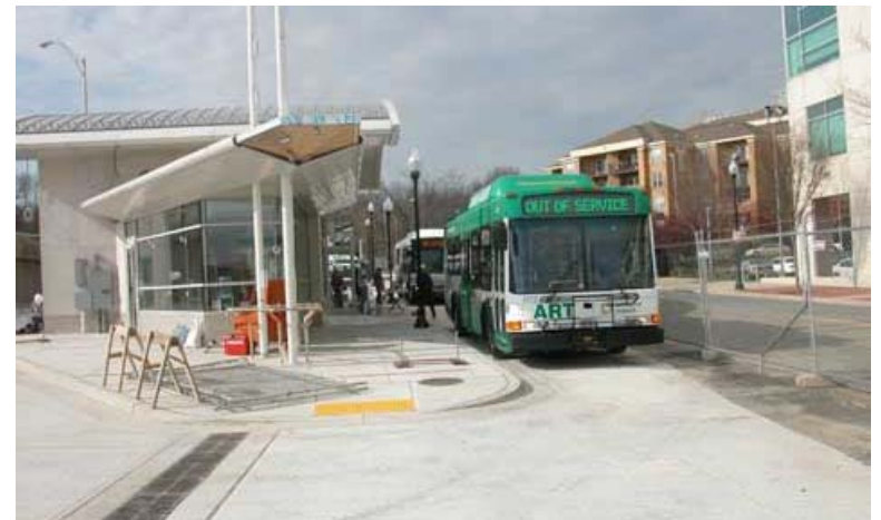
The Shirlington Transit Station, currently under construction in Arlington, VA.
