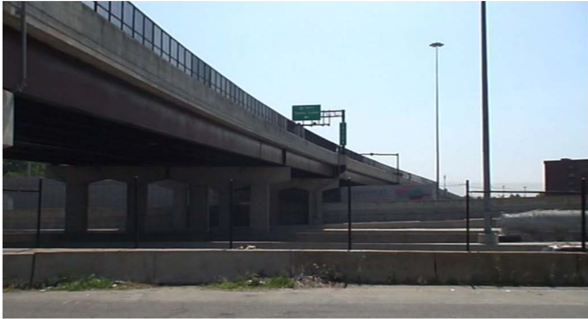
Looking East from potential site looking east at 95-495 southbound traffic.
