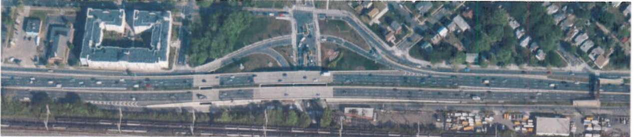
Photo Set One: This pair of photographs show the reconfiguration of the Nannie Helen Burroughs Ave NE interchange between 2005 and 2011. Note the lengthened deceleration lane to the right side of the 2011 image.
