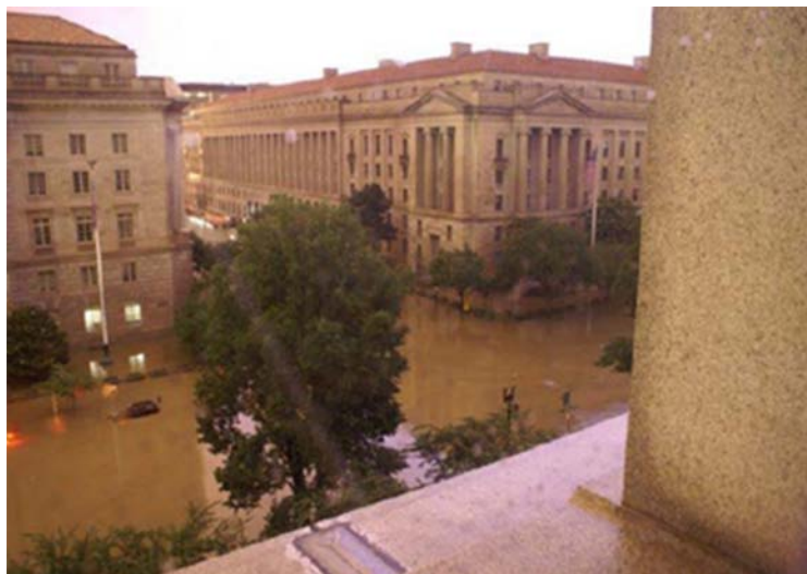
FIGURE 7: Flooding of Federal Triangle Area from the June 24-26, 2006 storm (Federal Triangle Stormwater Drainage Study, Greeley and Hansen, 2011)
