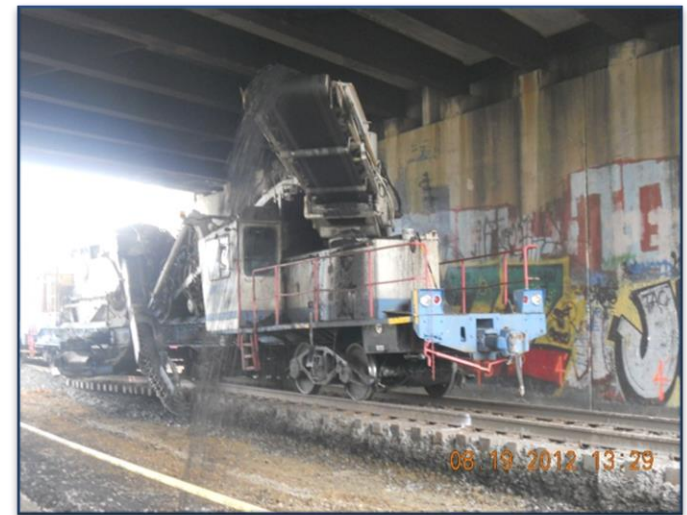
Track Lowering During Construction
