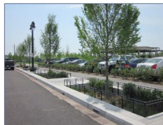
Bioretention with tree planter: District of Columbia
