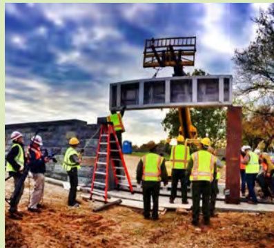
17th Street, NW Levee Installation Photo Credit: U.S. Army Corps of Engineers Baltimore District
