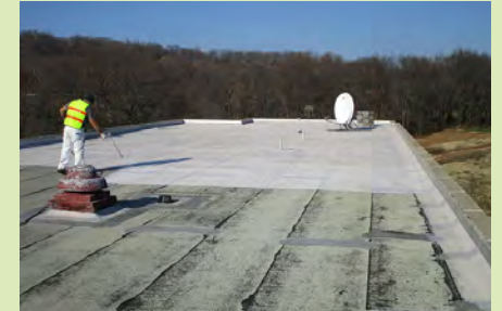
Crews install a cool roof at Browne Education Campus Photo Credit: Paul Lanning, Lightbox Energy
