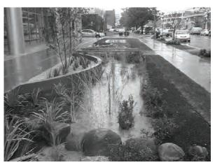
Rain gardens collect and filter stormwater runoff from paved surfaces like sidewalks and roads.
