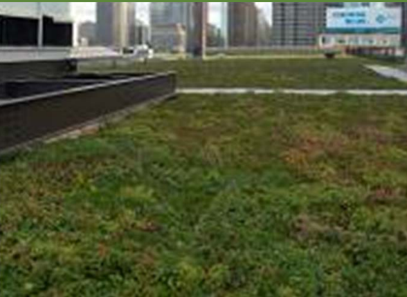
PECO Building, Philadelphia, PA
