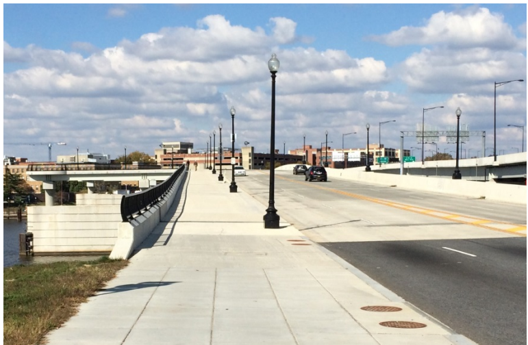
Figure 10: 11 th Street Bridge
