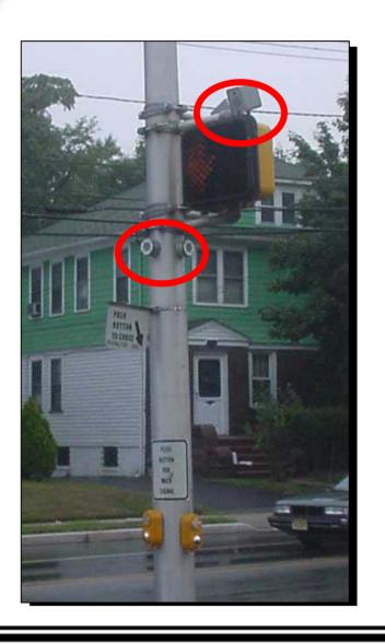
Locator tone speaker in this installation is mounted on pole; **WALK** indication comes from speaker above the pedhead, rather than at pushbutton
