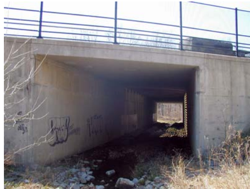
11 Photo A2.1. Wildlife Crossing in Fairfax County, Virginia.
