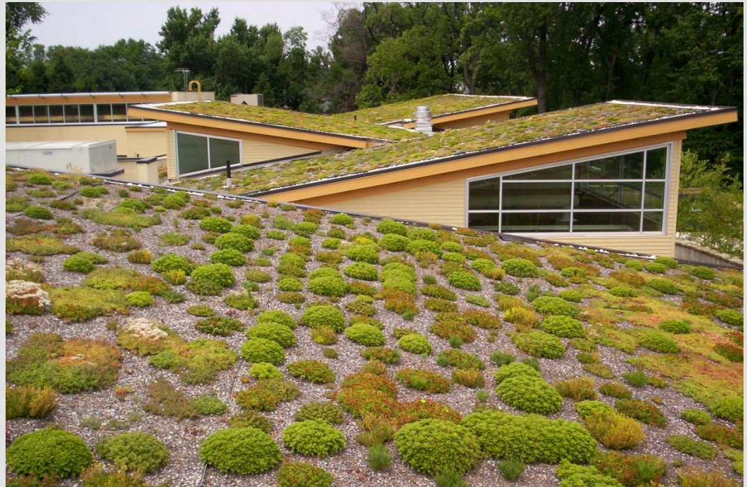
Green Roof at Walter Reed Community Center Photo Credit: Arlington County
