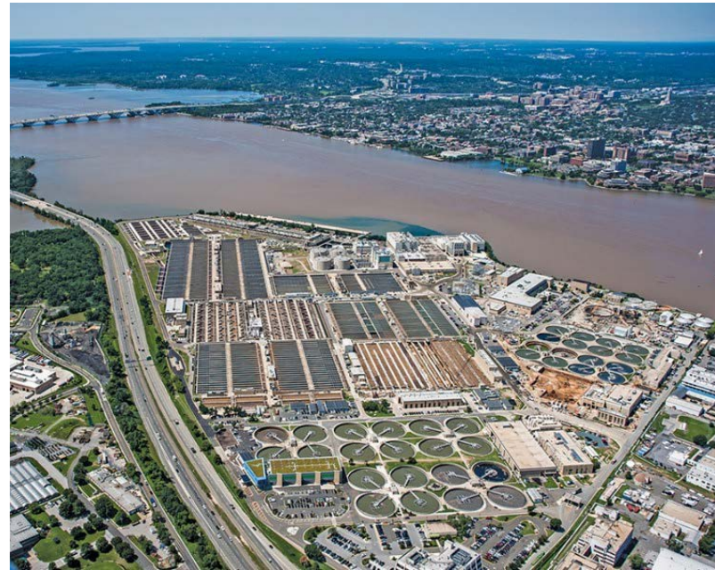
Blue Plains WWTP
