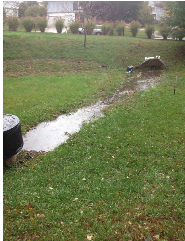
Figure 8 - College Hills pond facing northeast from the outlet towards the inlet. Direct flow path during storm event is evident.
