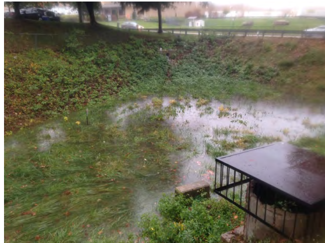
Figure 12 - McCormick Warehouse pond during storm event. Facing southeast from outlet towards inlet A.
