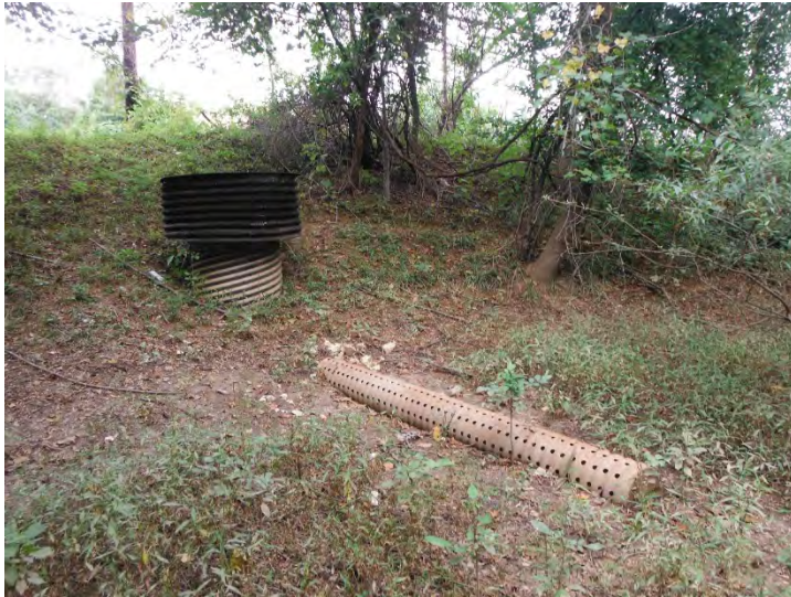
Hunt Ridge: Riser/low flow outlet pipe
