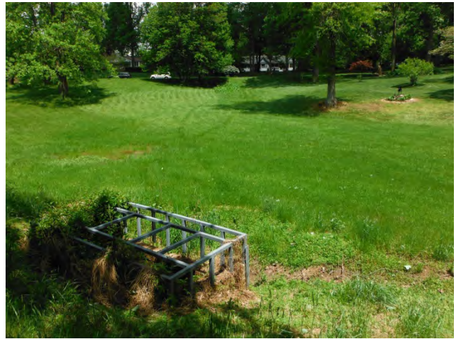
Figure 10 - Fields of Harvest pond overview facing north from the outlet towards the inlet.
