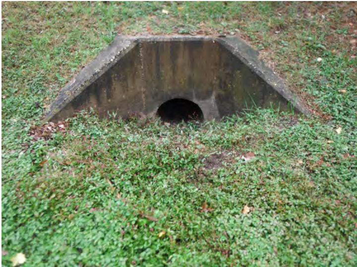
College Hills: Inlet prior to pilot channel excavation
