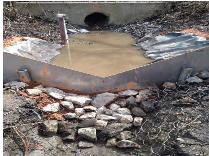
Glyndon: Inlet A immediately following weir installation
