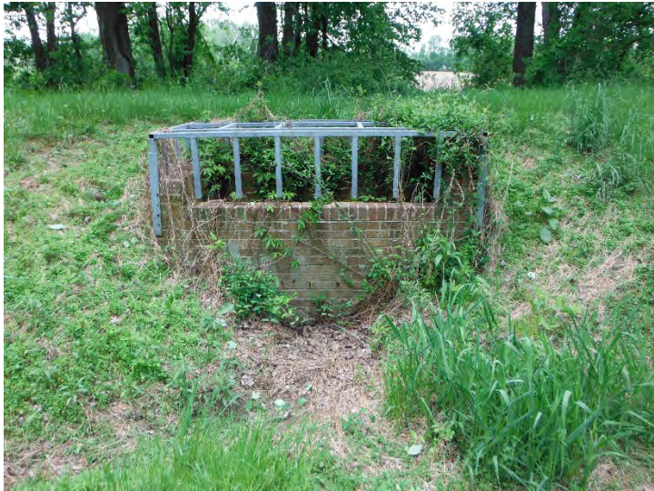
Fields of Harvest: Outlet box structure, low flow orifice obscured by vegetation
