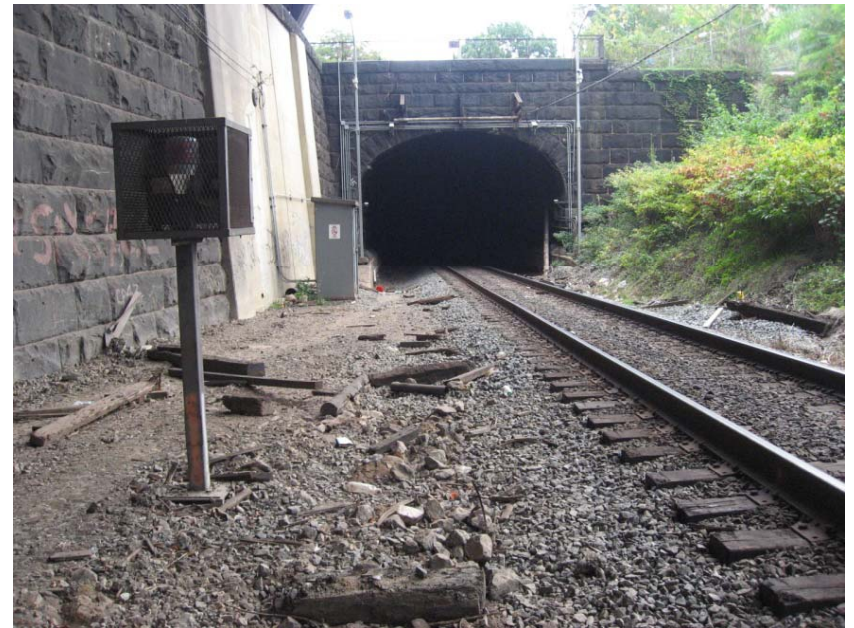
CSX Virginia Avenue Tunnel (West View)
