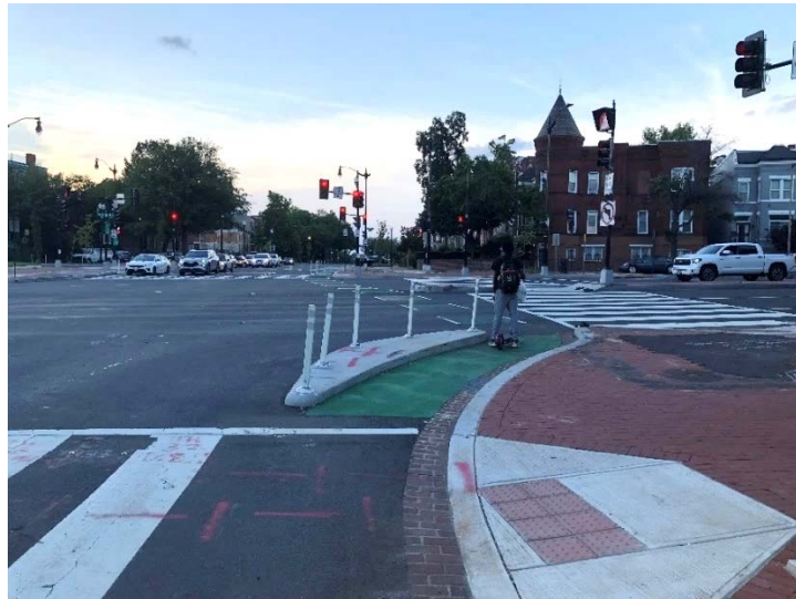
Figure 31: Partial Protected Intersection/TPB/Michael Farrell
