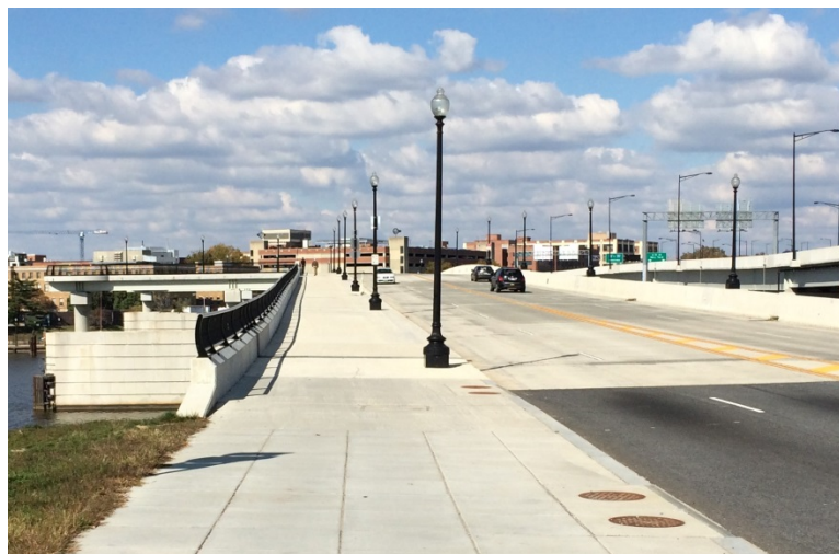
Figure 37: 11th Street Bridge/TPB/Michael Farrell
