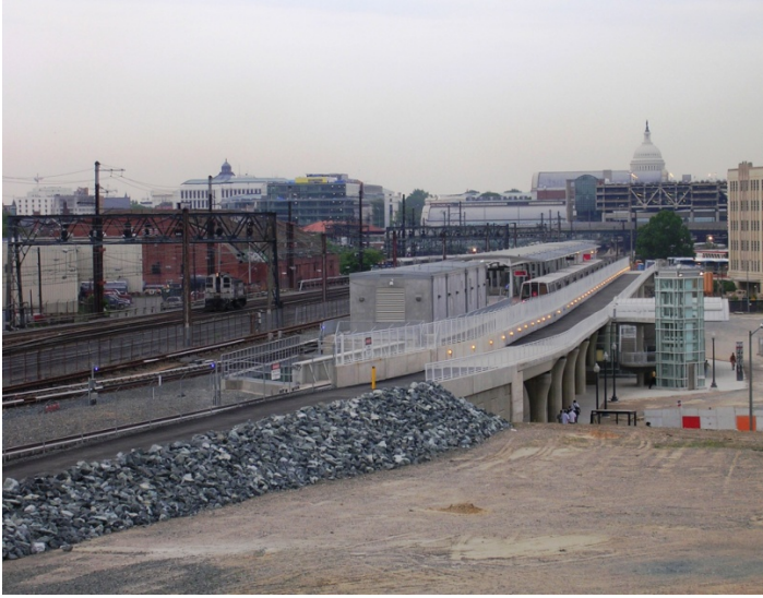
Figure 2: NOMA/Gallaudet Metro Station and Metropolitan Branch Trail/TPB/Michael Farrell
