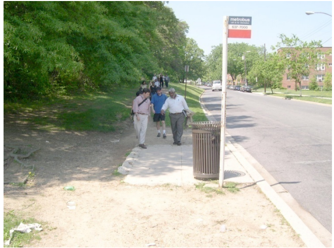
Figure 6: Missing Sidewalk/TPB/Michael Farrell
