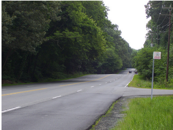
Figure 58: Lawyers Road Before Road Diet/VDOT
