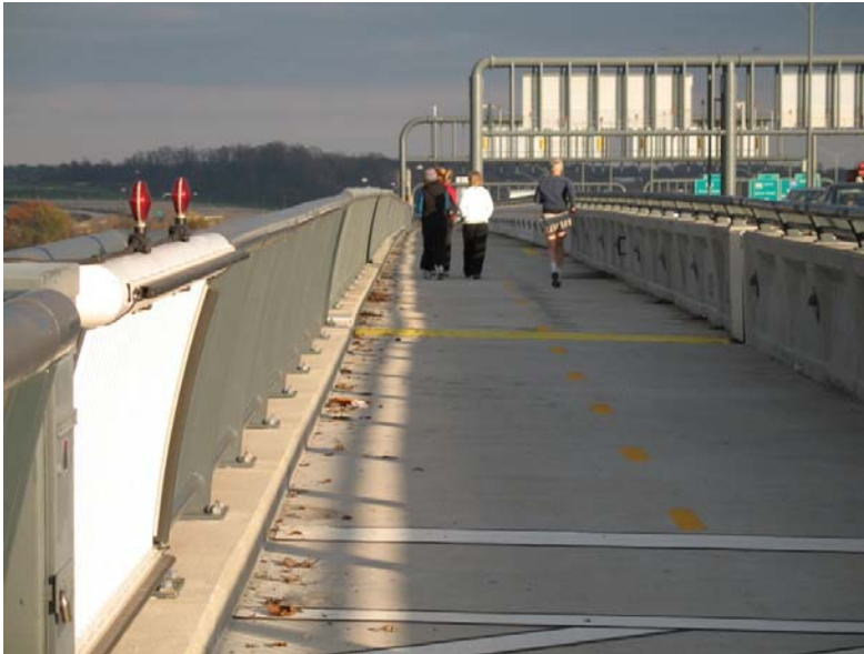
Figure 2: Woodrow Wilson Bridge Trail
