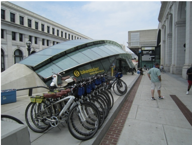
Figure 15: DC Bike Station at Union Station Photo Credit: COG/TPB
