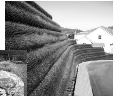
Vegetated retaining wall (Denbow.com)
