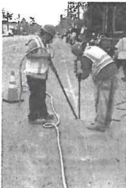
Magnet installation.
