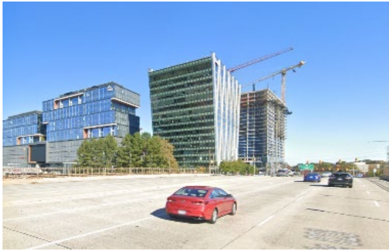
Current configuration of Wiehle Ave over Dulles Toll Road
