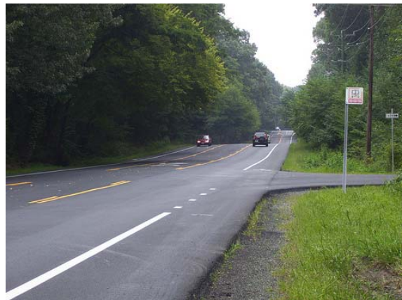
Figure 59: Lawyers Road After Road Diet/VDOT
