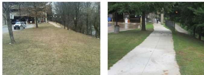
FRANCONIA - SPRINGFIELD BEFORE AND AFTER, NEW SIDEWALK TO IMPROVE SAFETY
