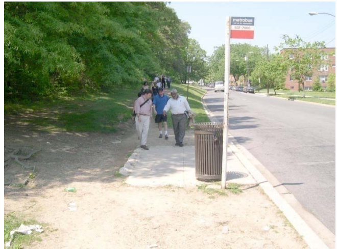
Figure 6: Missing Sidewalk/TPB/Michael Farrell
