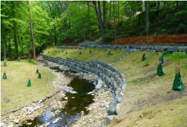
Windy Run, After Restoration
