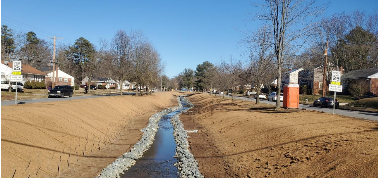
Briers Mill Run, After Restoration
