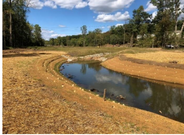
Dewey Creek, After Restoration
