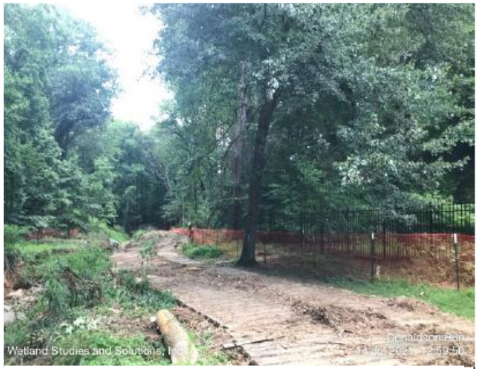
Example of saving trees during construction of the Donaldson Run Tributary B Stream Restoration Project in Arlington County. Access to the site was adjusted to save a tree important to the landowner. (Wetland Studies and Solutions, Inc.)
