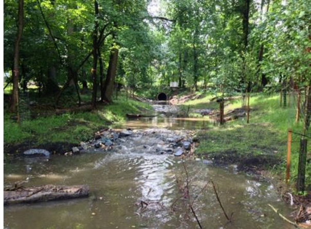
Brewwood Tributary, After Restoration
