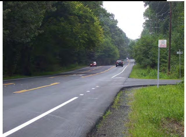
Figure 10: Lawyers Road After Road Diet
