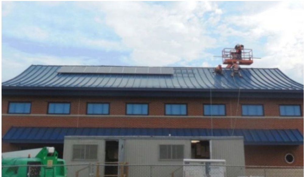
Installation of solar panels at Metro's net zero energy stormwater facility.
