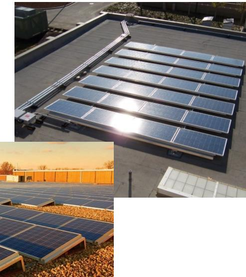
Example: Low-Tilt, Ballasted Racking System
