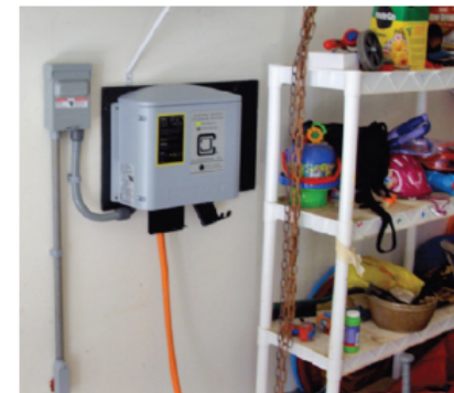
Figure 1. A typical wall-mounted Level 2 home charging station inside a garage. Photo courtesy of Clean Fuel Connection, Inc.
