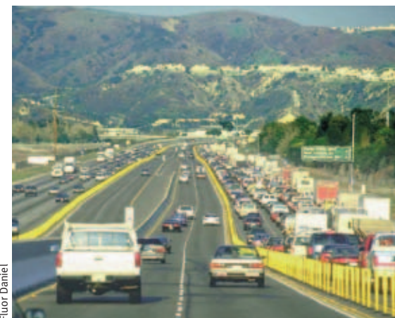
HIGH OCCUPANCY TOLL (HOT) LANES PERMIT SOLO DRIVERS TO PAY TOLLS TO USE CARPOOL LANES. THE HOT LANE FACILITY PICTURED BELOW IS IN ORANGE COUNTY, CALIFORNIA.
