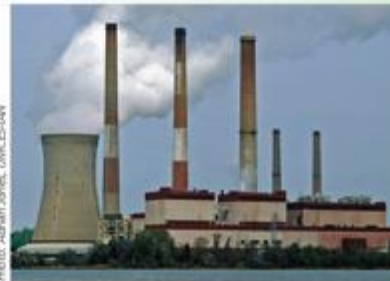
Chalk Point Power Plant on the Patuxent River.
