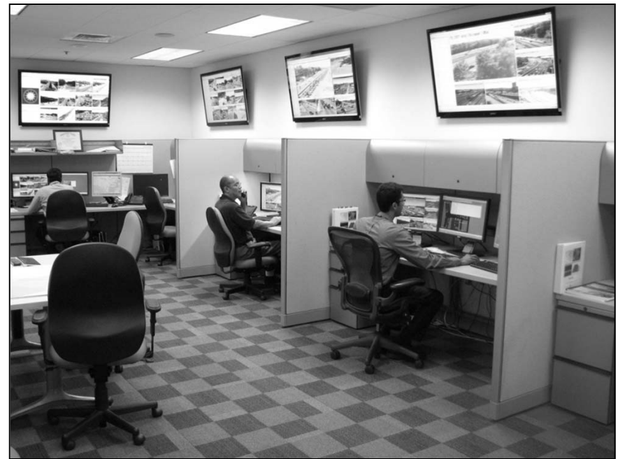
Signal Operations Center (SOC)
