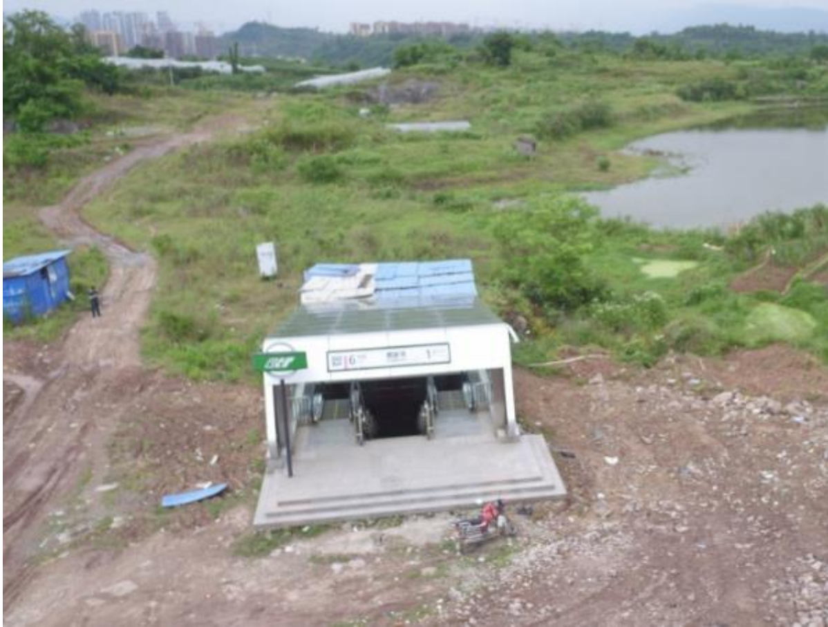
Caojiawan Station, Chongqing
