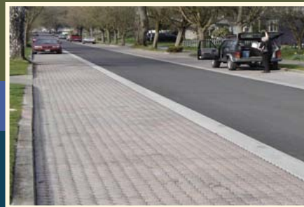
Permeable interlocking concrete pavement (PICP) in parking lanes
