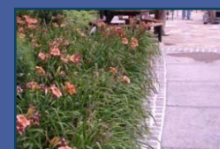
Bioretention next to pervious concrete with recycled materials for edges
