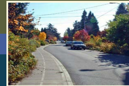
Curb bump outs/extensions provide bioretention areas; traffic calming measures improve safety
