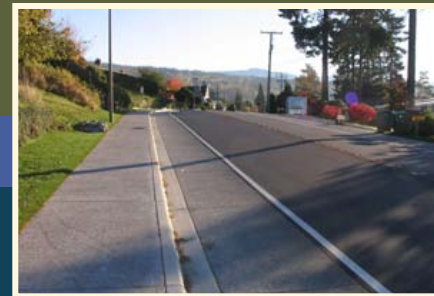
Streets constructed of pervious concrete pavement or other permeable surfaces
