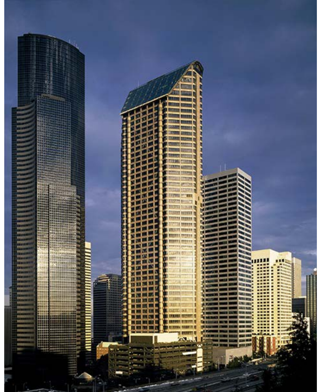
Seattle Municipal Tower, a 62-story office building studied in the Urban Freight Lab
