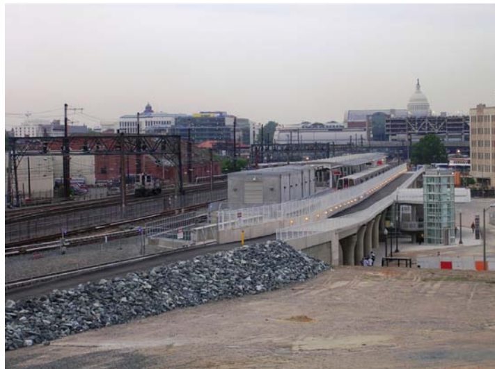
Figure 3: New York Avenue Metro Station and Metropolitan Branch Trail
