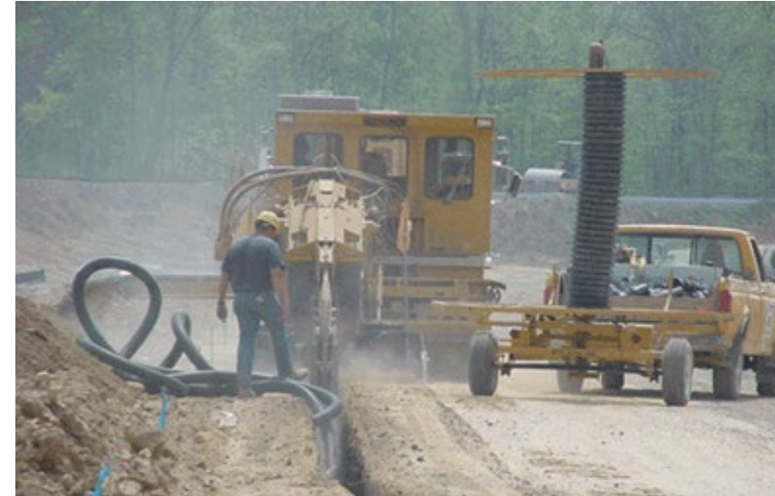
Underdrain installation. Source: Ohio Department of Transportation
