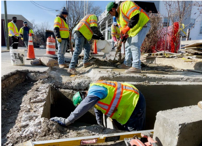
A crew pours concrete to form the catch basins for the new, wider inlets on Hume Avenue.
