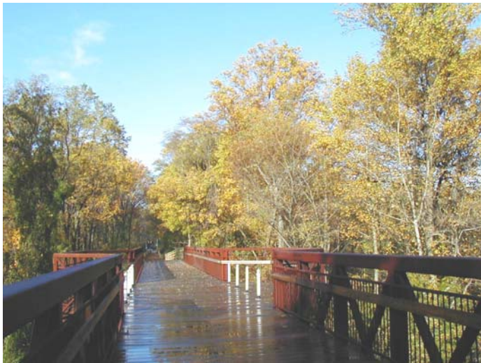
The Capital Crescent Trail Bridge over Rock Creek, Chevy Chase, MD opened in 2003
