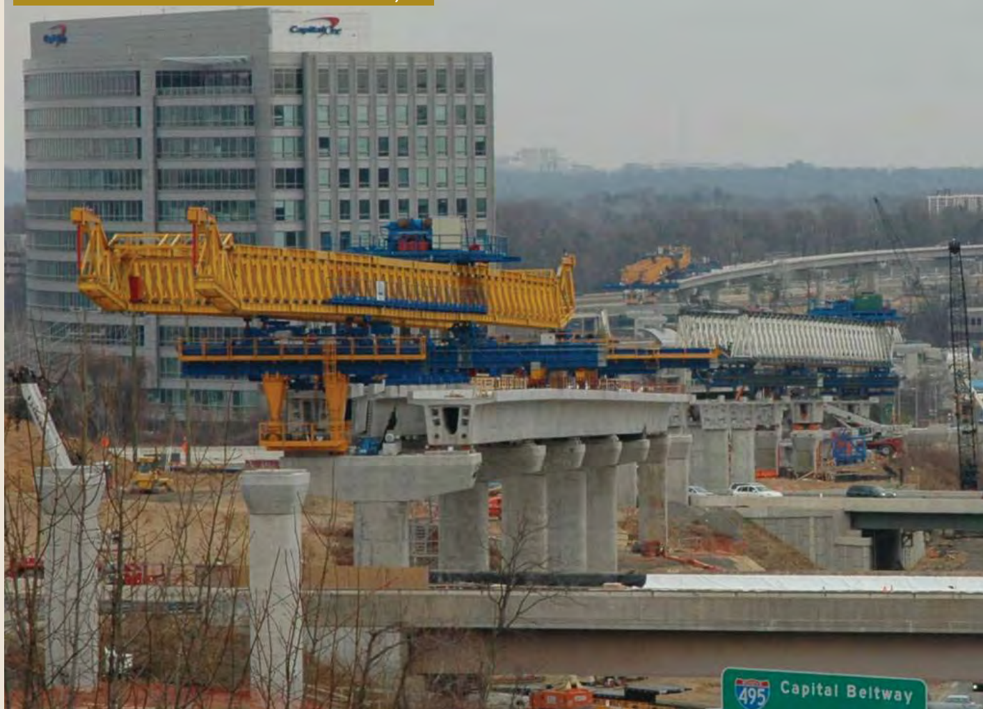
Construction of the Dulles Corridor Metrorail Project
