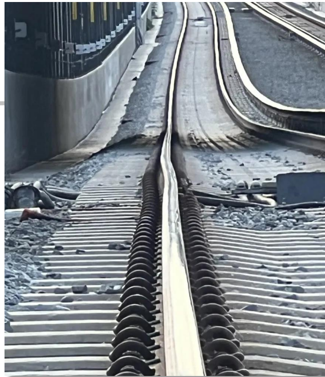
Heat kink in MetroRail line near Crystal City stop, summer 2024. Source: X
