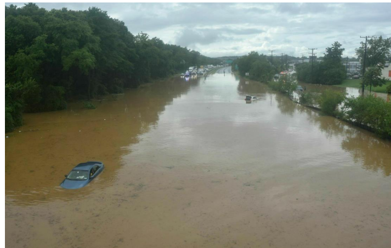
Route 50 in Prince George's County flooded after heavy rains in 2020. Source: WTOP News.
