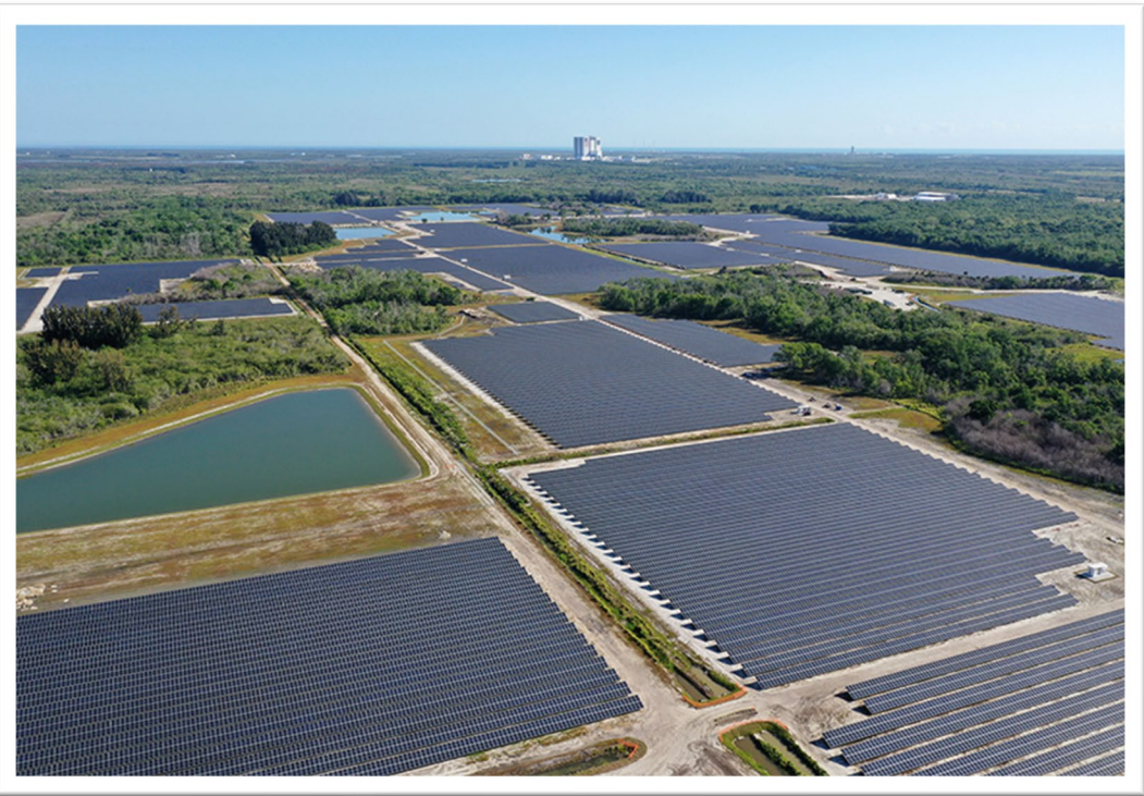
UTILITY-SCALE SOLAR FACILITY AT KENNEDY SPACE CENTER IN FLORIDA
