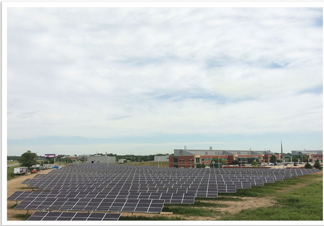
COMMUNITY-SCALE SOLAR FACILITY IN KALAMAZOO, MICHIGAN
