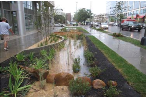
Rain garden: District of Columbia
