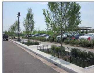
Bioretention with tree planter: District of Columbia
