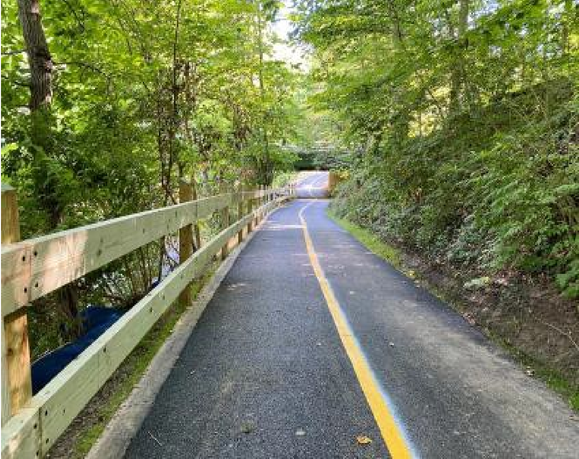
Porter Street Underpass in Rock Creek Park (Joe Flood/ Flickr )
