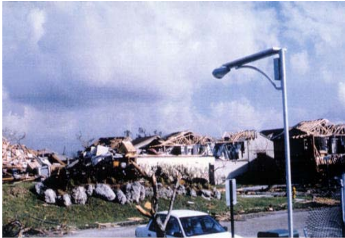
After Hurricane Andrew, Picture facing N.W.
