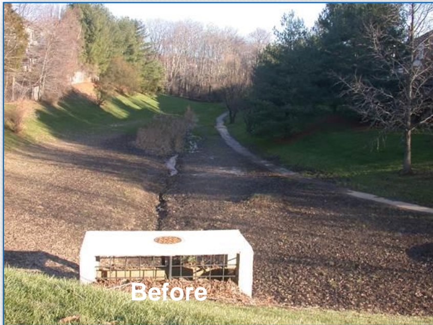
Fallsberry Stormwater Management Pond in Potomac, Maryland
