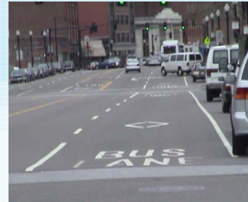
Middle Lane Reservation (Cleveland, Ohio)
