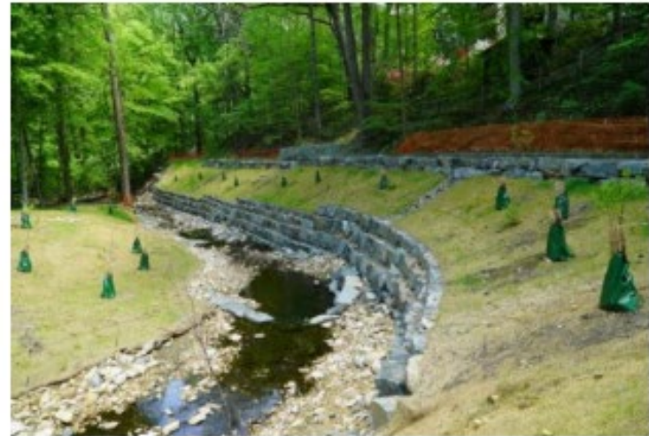
Windy Run, After Restoration
