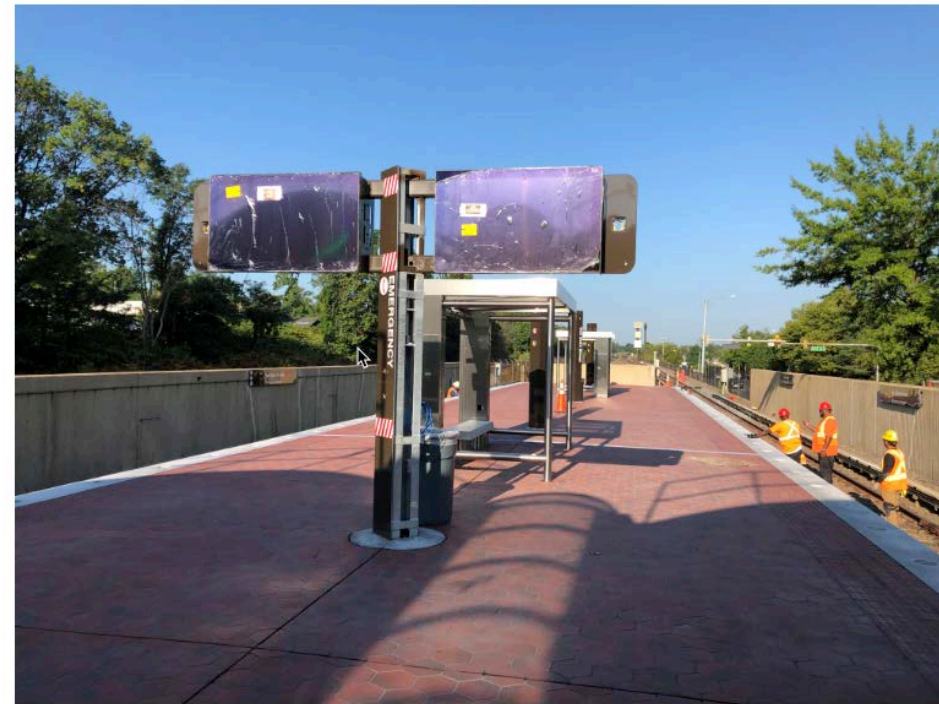
Van Dorn St - PID screens installed
