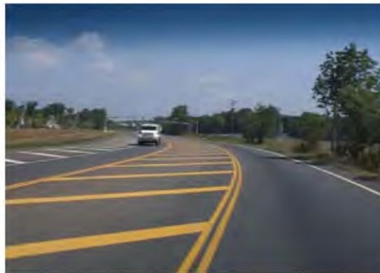
Route 606 Looking North Approaching Overland Drive
