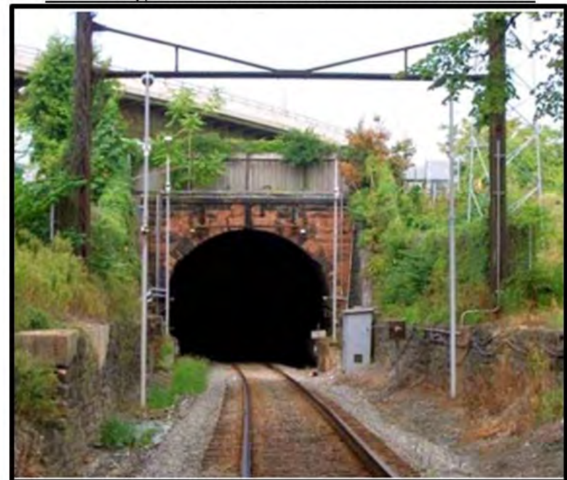
CSX Virginia Avenue Tunnel West Portal View
